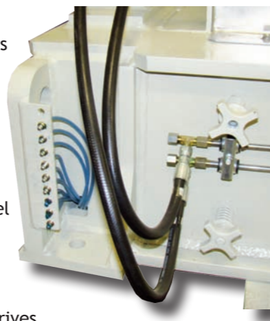
View shows the grease manifold and scraper tension adjusters
